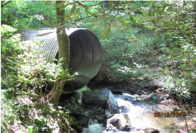
Bryant Creek crossing (FS Road 33A) before replacement – outlet view of round culvert creates barrier to aquatic movement and impacts stream channel.
