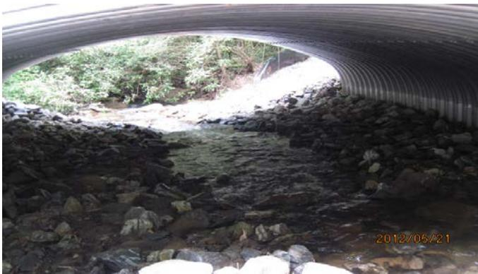
Bryant Creek crossing (FS Road 33A) after replacement – inlet view of arch culvert – removes barrier, restores natural channel.
