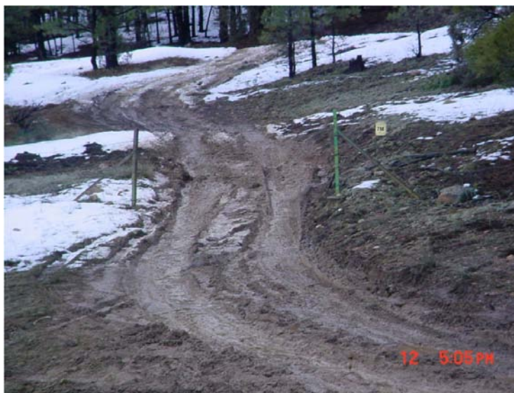
Figure 28. Soil damage from vehicle use on wet soils during hunting season in game management unit 11M
