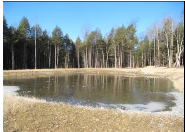
2 nd - Water enters the first pond (aerobic limestone basin) where it flows through limestone and begins chemical reactions that will neutralize its acidity.
