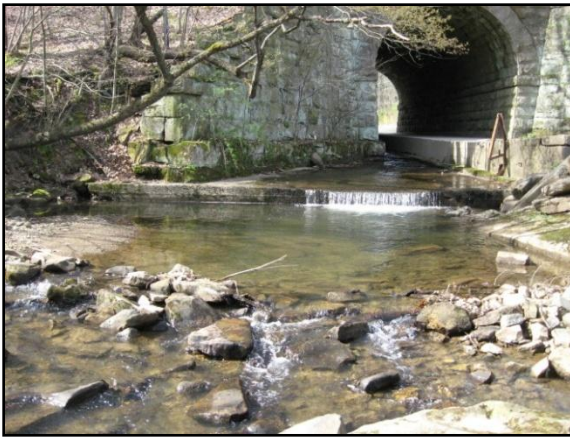
Morrison Run before and after construction of an engineered rock ramp designed to facilitate aquatic organism passage through a historic railroad viaduct
