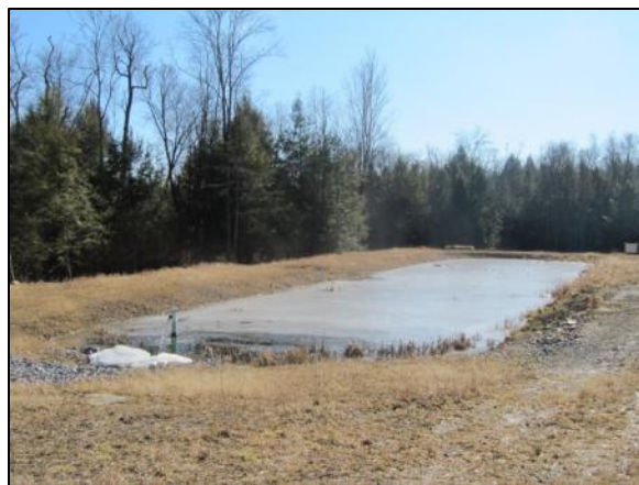
3 rd - Partially treated water flows into a second pond (anaerobic vertical flow wetland) lined with limestone and a mushroom compost substrate, where additional alkalinity is generated through dissolution and bacterial sulfite reductions.
