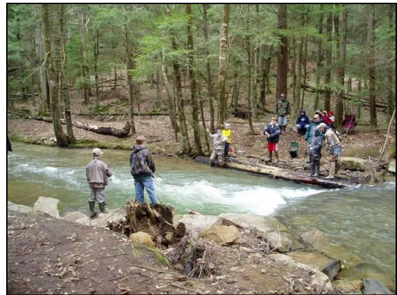
Log devices placed in Ross Run to provide pool and overhead cover habitat
