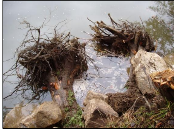
Root wads placed in Spring Creek
