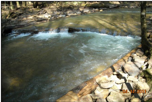
Log devices placed in Ross Run to provide pool and overhead cover habitat
