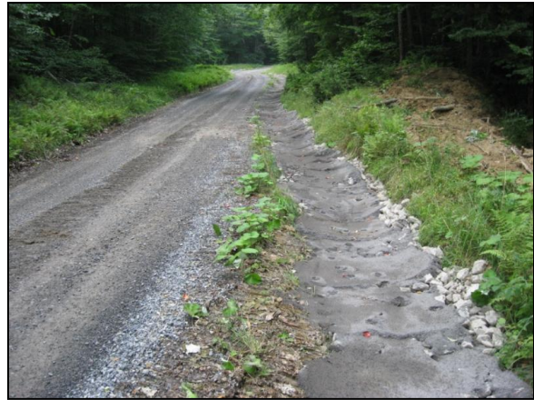
Alkaline road runoff channel in road ditch lines along Forest Road 279 to supply buffering capacity to tributaries of South Branch Kinzua Creek.
