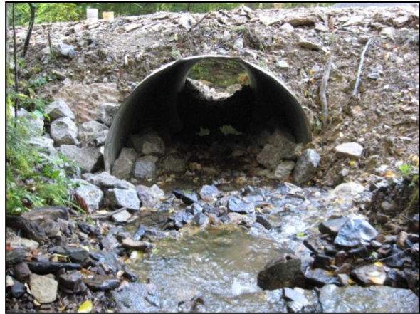
Aquatic organism passage restored on a tributary to SBKC
