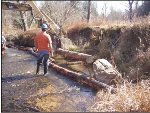
Construction of Modified Mudsills
