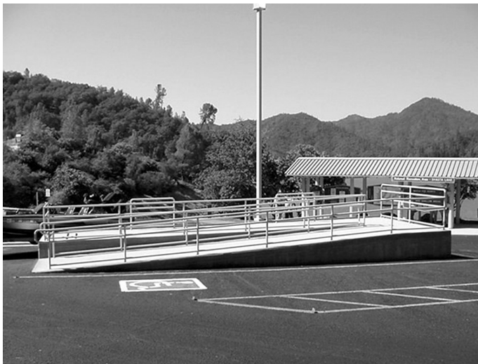
Accessible loading platform located at the Packers Bay public boat ramp at Shasta Lake.
