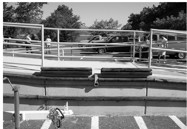
Patient lift receiver on accessible loading platforms.
