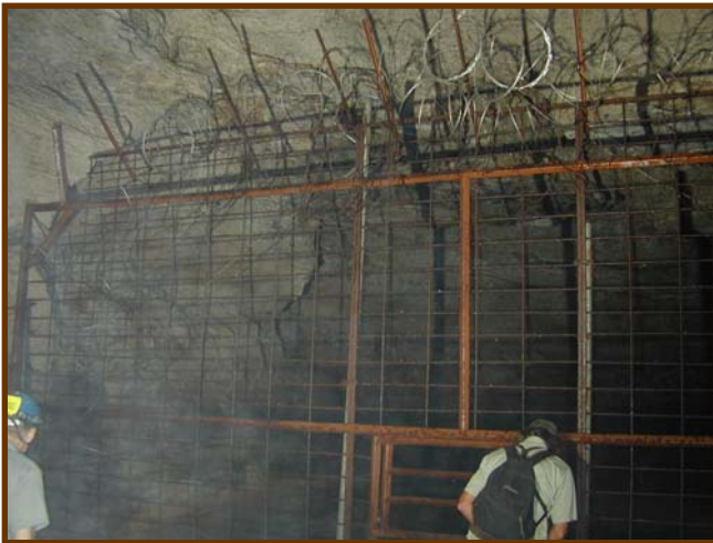
Bat Cave – Ozark County- gate inspection
