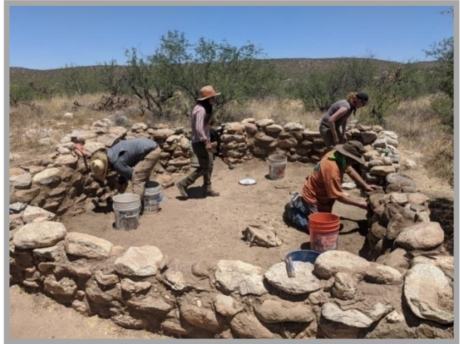
Figure 15. Coronado National Forest Heritage team and volunteers collaborating to stabilize the remains of historic Romero Ranch house. Photo courtesy of Maxwell Forton, USDA Forest Service.
