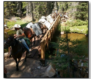
Newly rebuilt Ross Fork Bridge.
