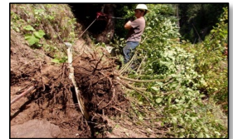
Trail crew using ground based rigging
