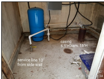
Timberlane pump house before and after repairs
