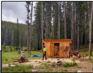
Removing a dangerous snow load from the Gordon Reese Cabin
