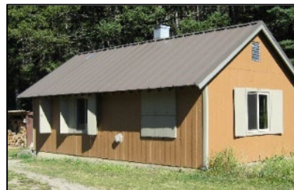
Dry wolf cabin upgrades
