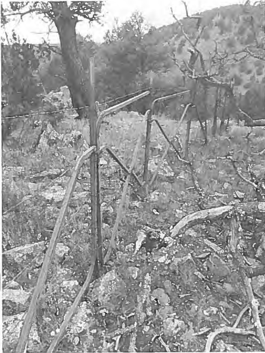
Southside brace with donwed tree on it
