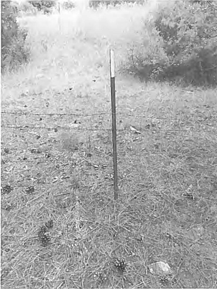
Reattach top wire after corner
