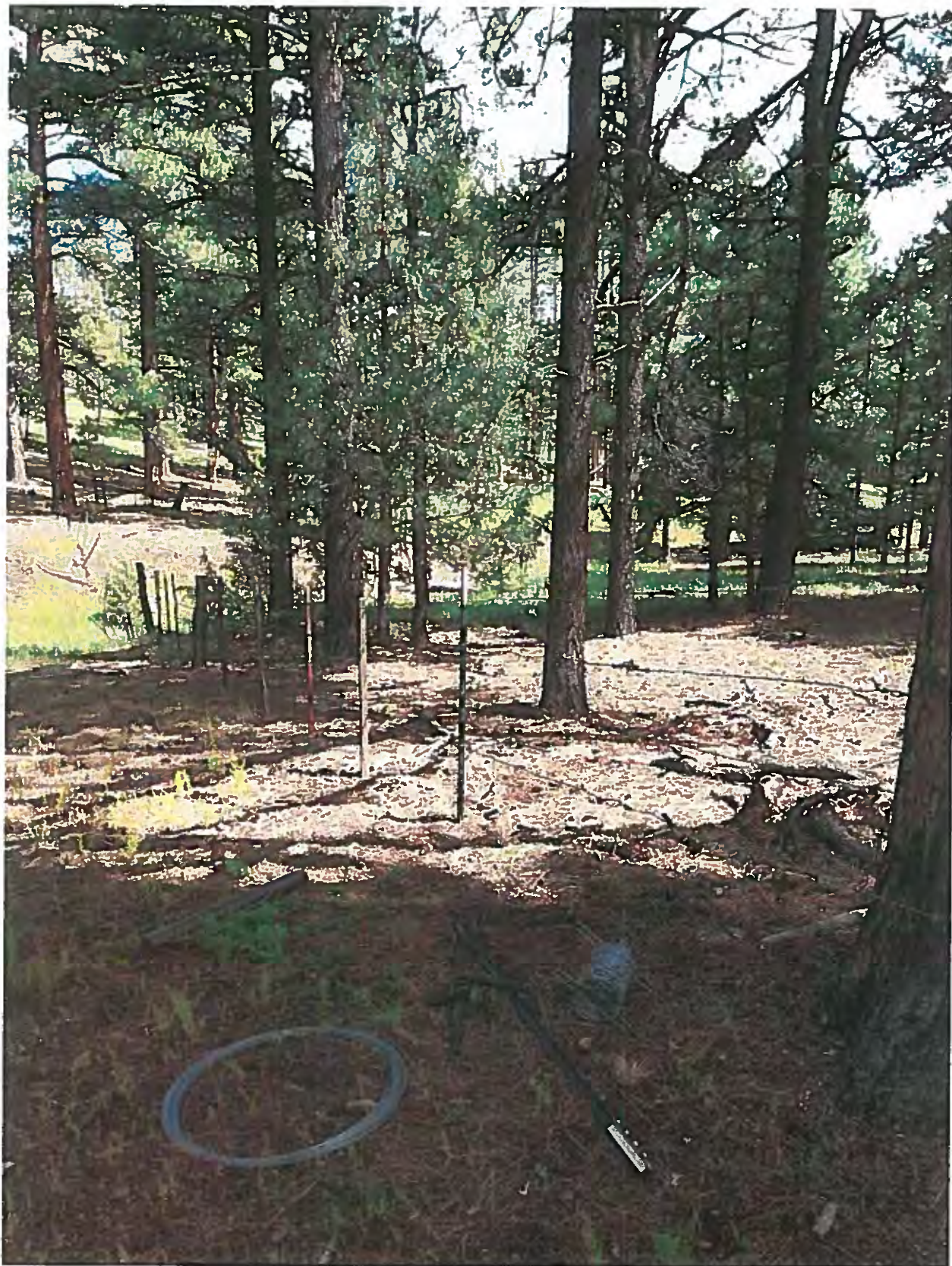
Figure 5 north side of northwest corner repaired.
