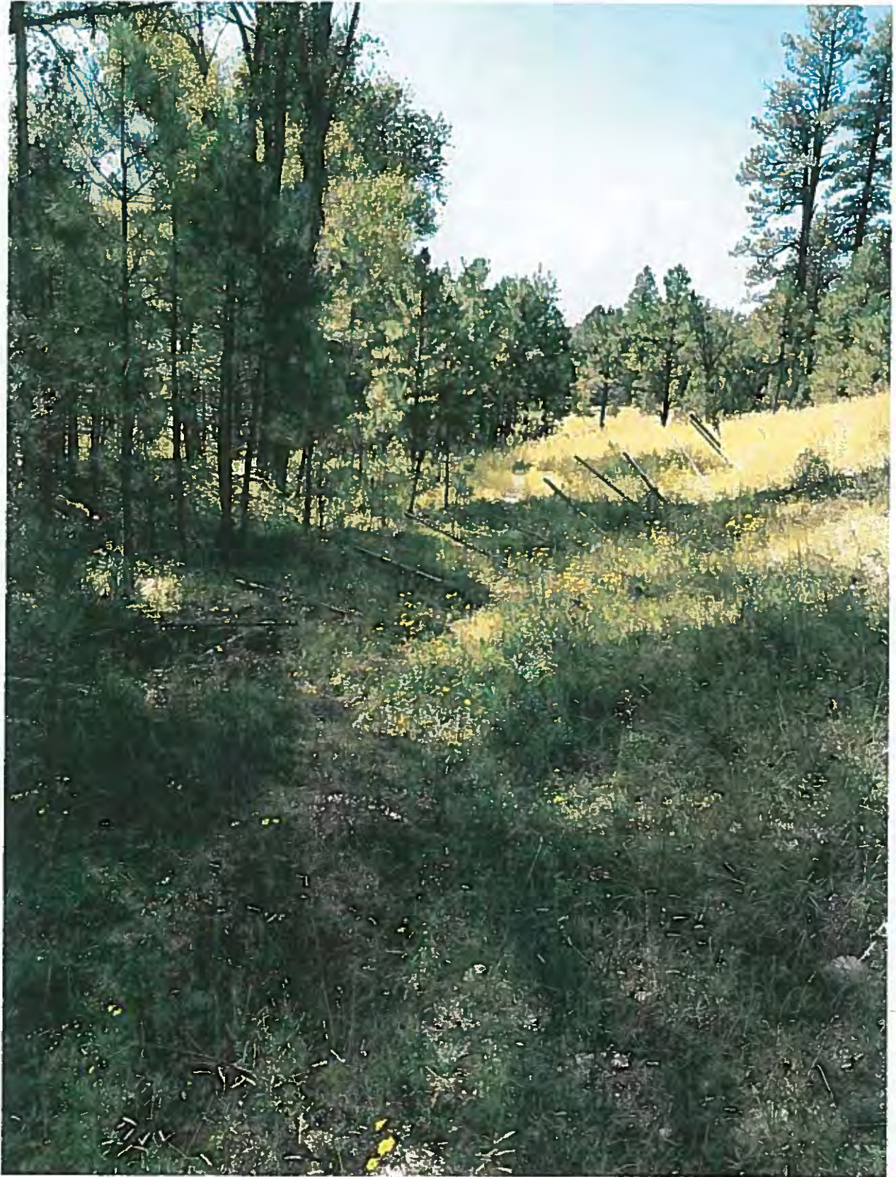
Figure 9 fence downed on west side of the south water gap.
