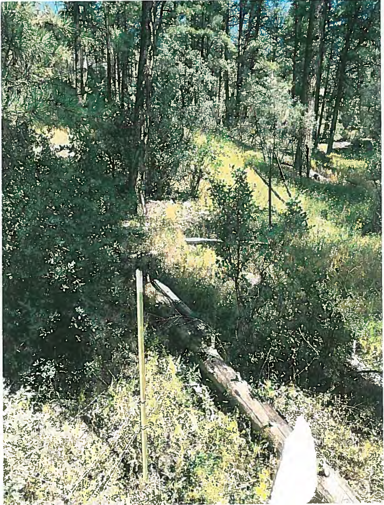
Figure 8 downed section of fence due to fallen tree
