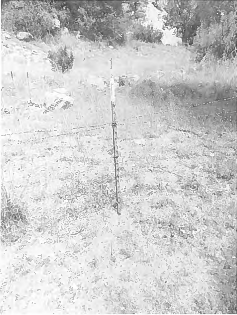
Twisted wire on north side
