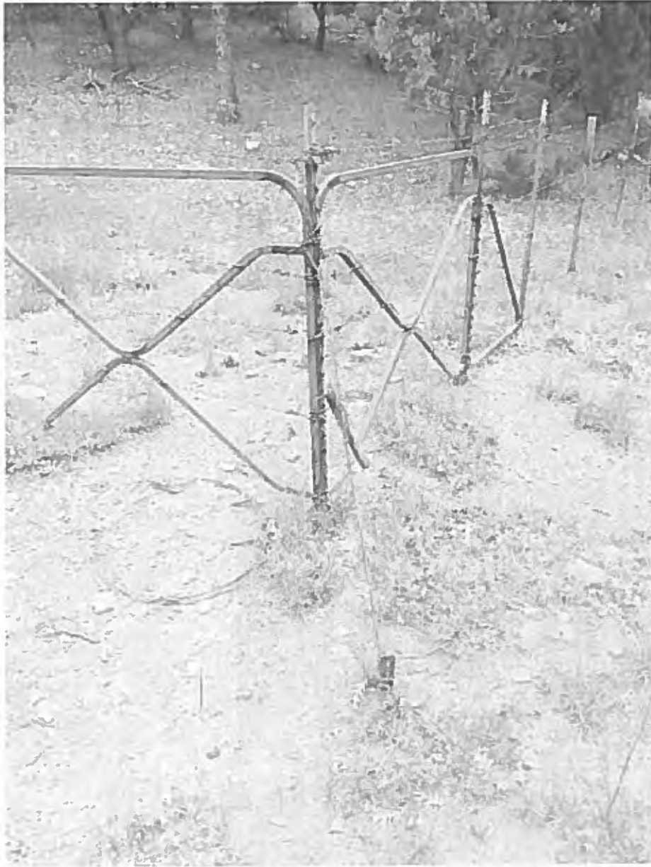
Corner brace on south side
