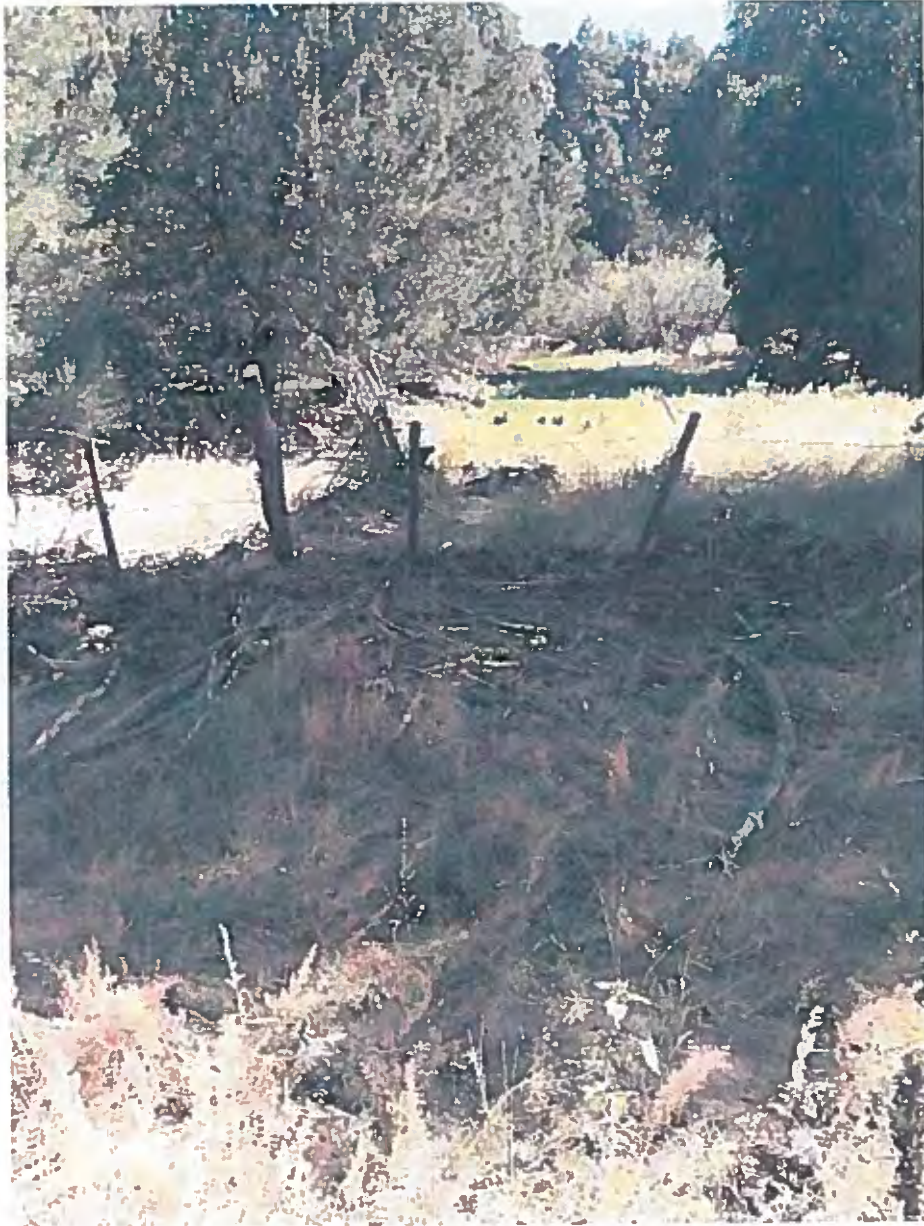
Secondary channel water gap fixed
