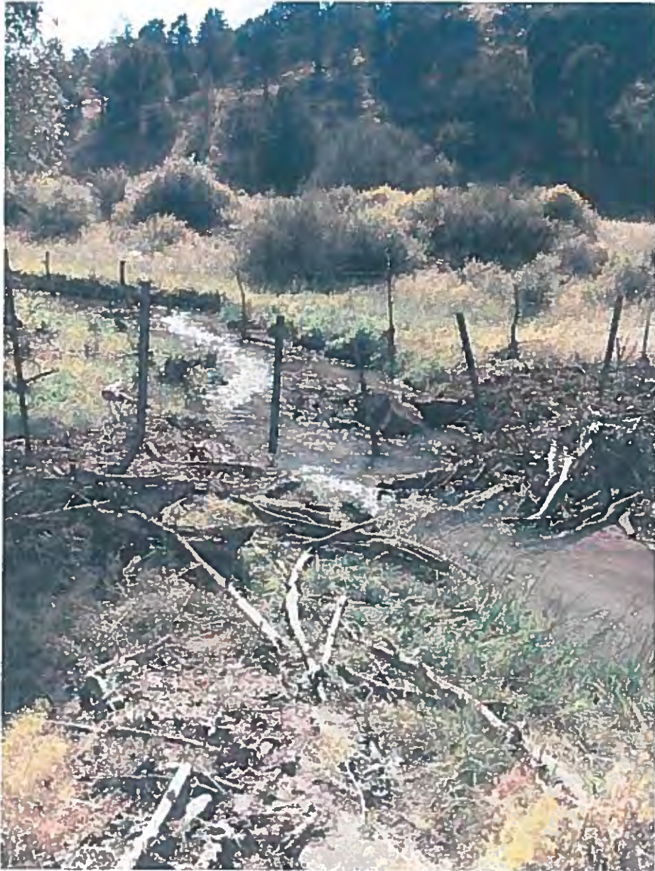
Water gap fixed
