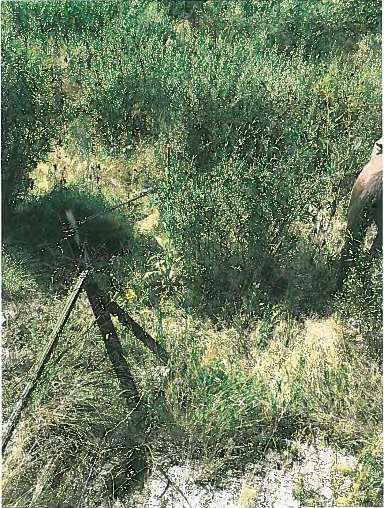
Figure 12 brace on east side of north water gap leaning but still functioning.
