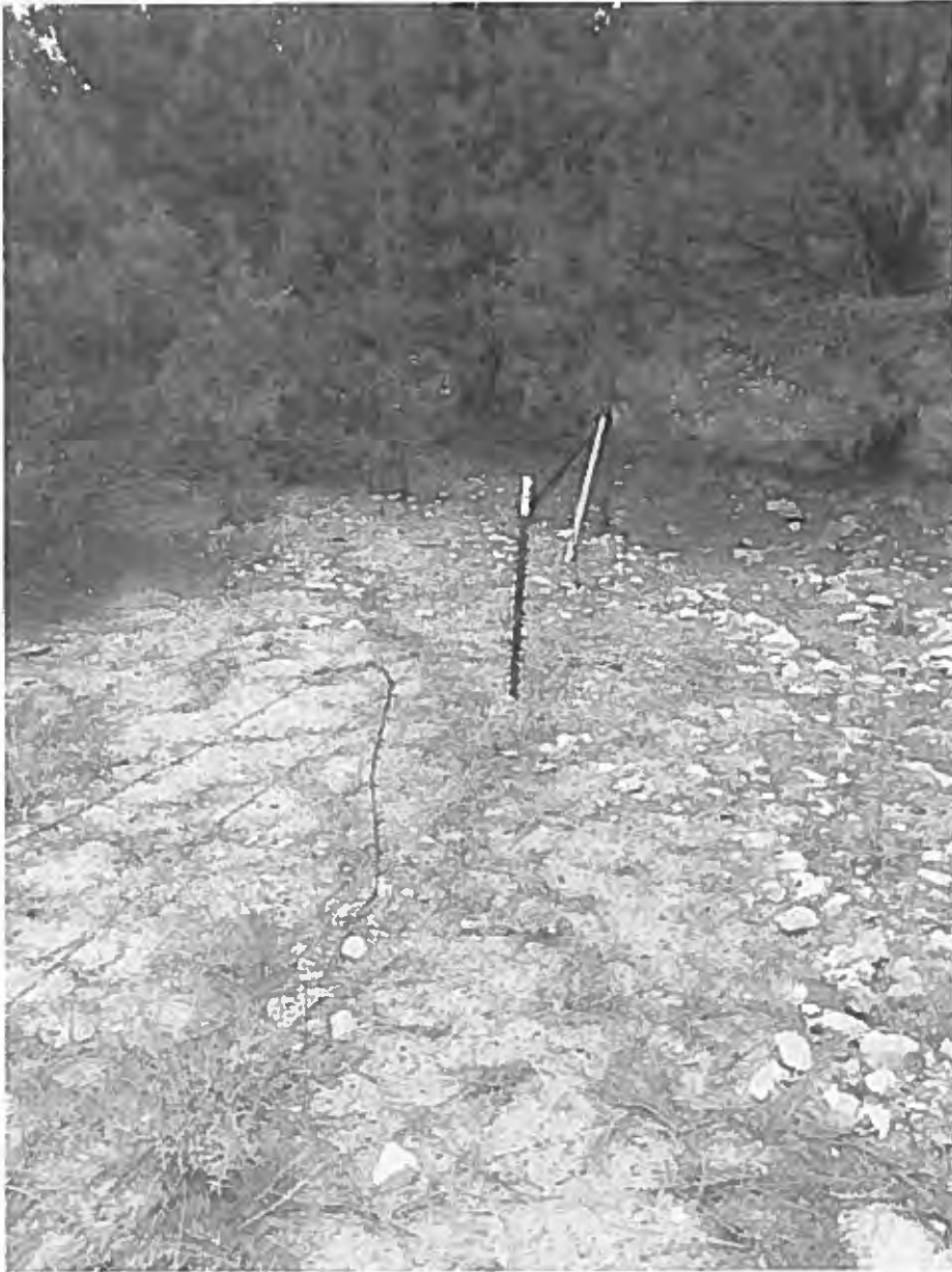
Top Wire tighten and new stays at corner of north side
