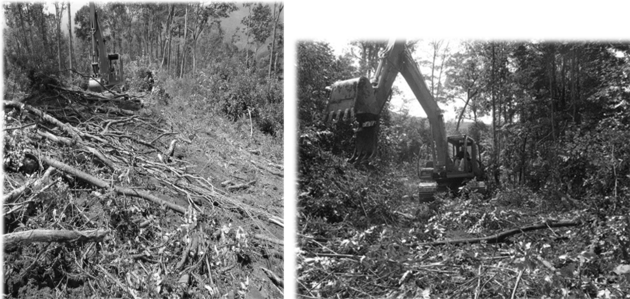
Figure 20. Farmers Branch Timber Sale in harvest unit 4 (left) and Eagle Fork Timber Sale unit 2 (right) subsoiling to reduce soil compaction and detrimental soil disturbance from skid roads and landings
