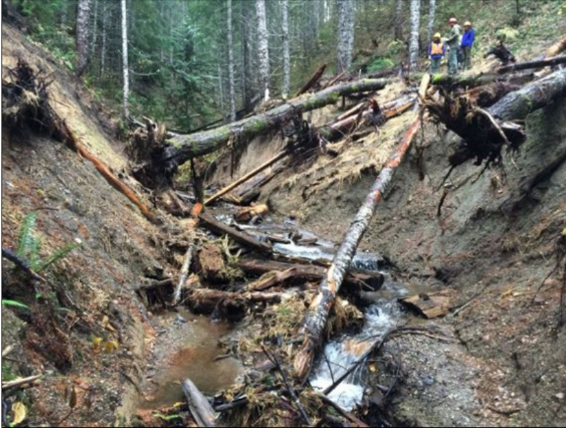
Photo 37. Road decommissioning on Gifford Pinchot National Forest
