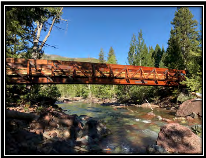
The new North Fork Cabin bridge was completed in 2019
