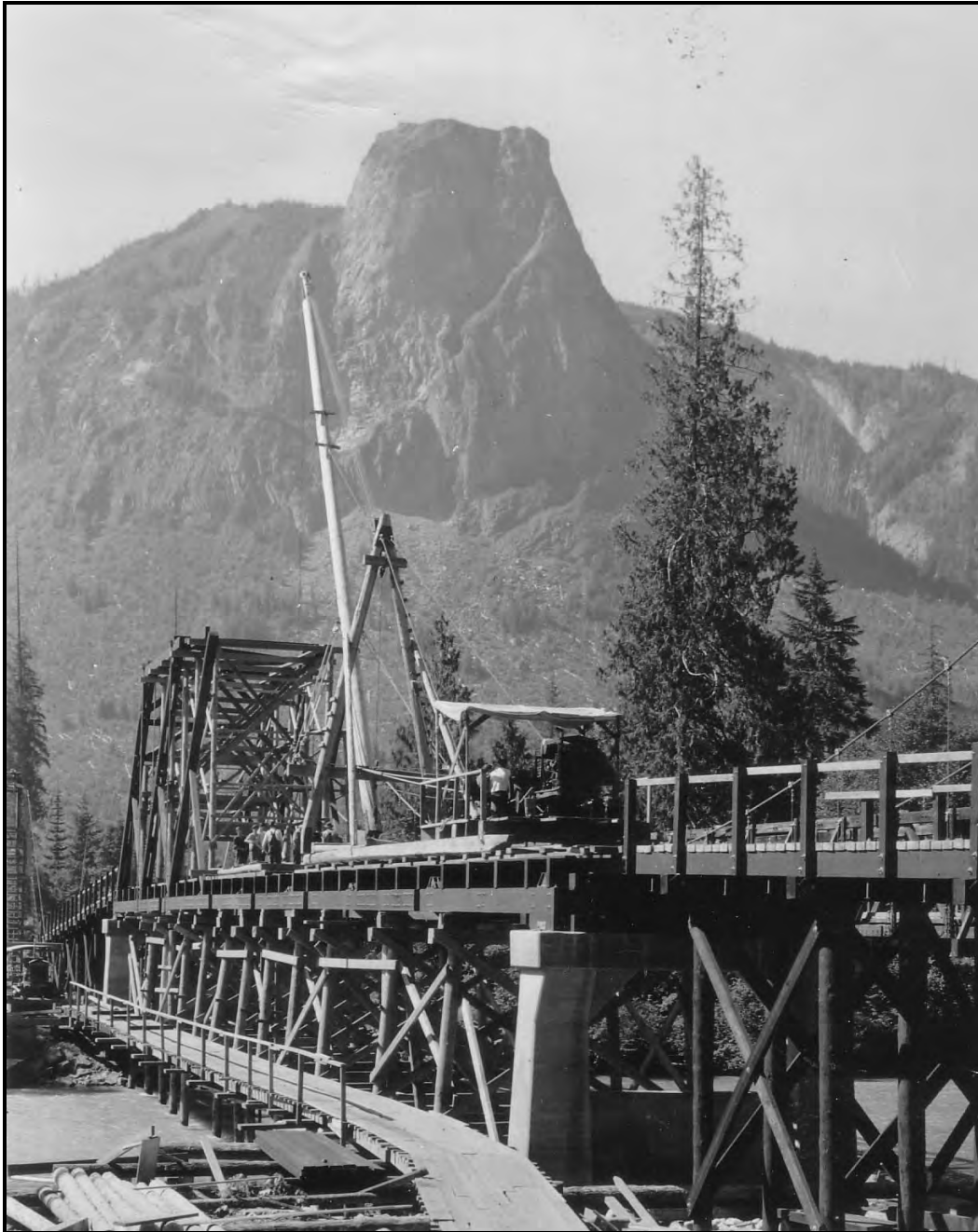
Cispus Valley Bridge under construction by the CCC in 1939, Tower Rock in background. The pile driver described by Mr. McMahan is visible in the center of the photo. The photograph is from the Gifford Pinchot National Forest archives.
