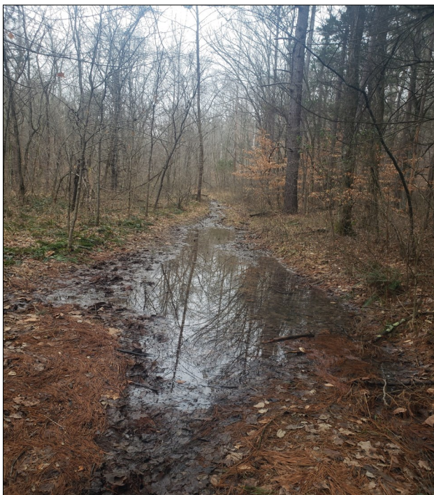
An entrenched forest road has trapped water run-off causing rutting and erosion issues.
