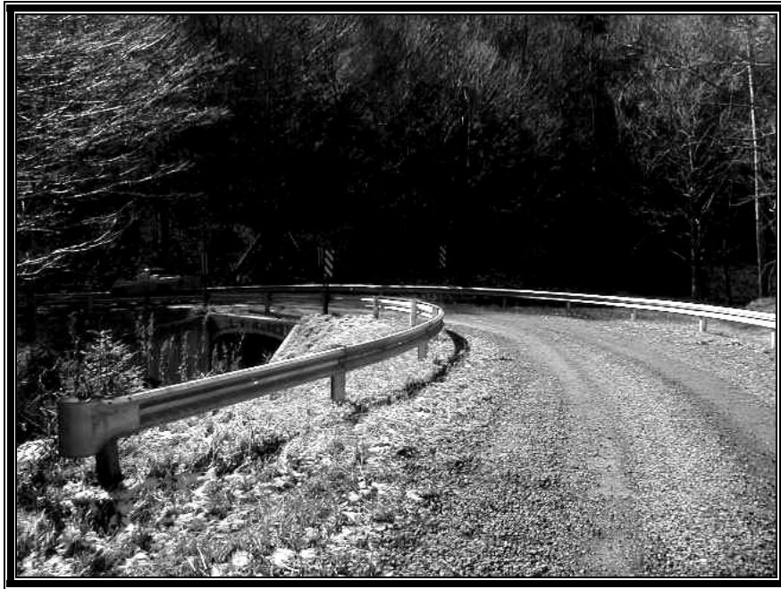
Forest Road – Maintenance Level 4
