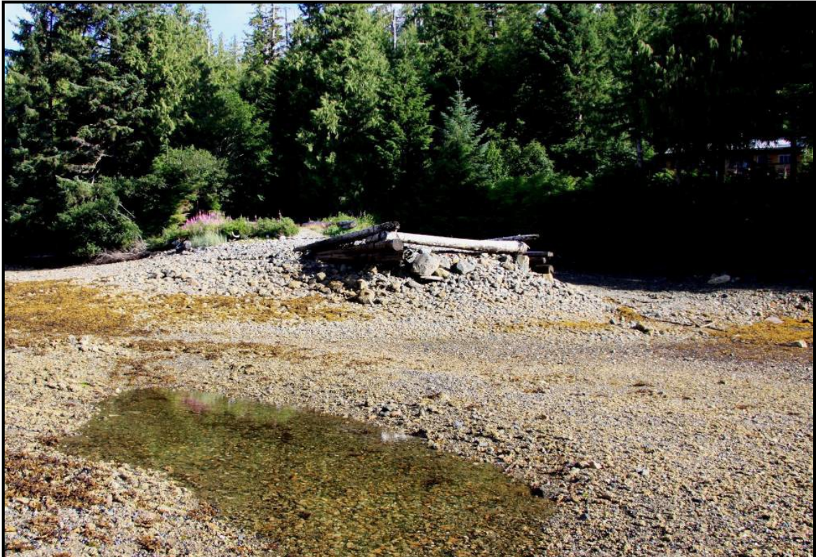
Photograph Looking North at the Older and Westernmost Rock Loadout Ramp
