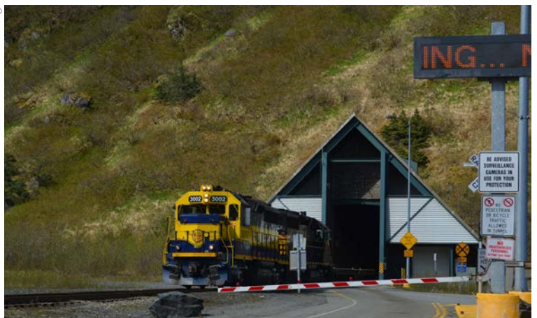
Whittier Tunnel entrance.
