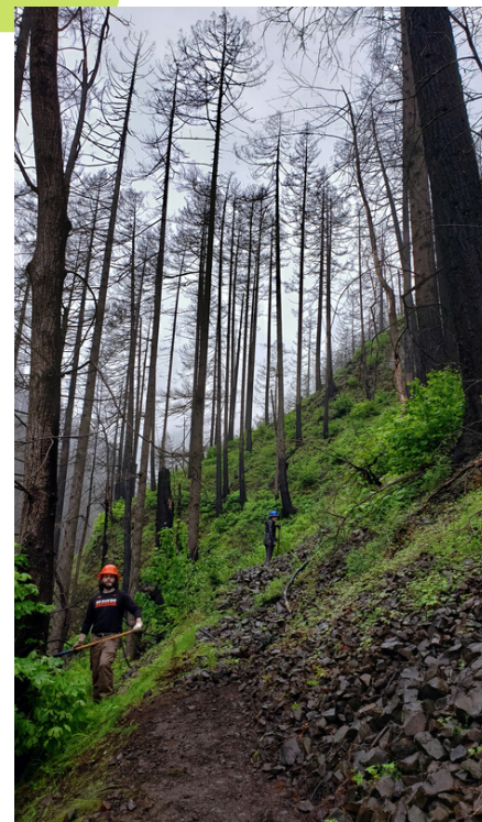
Showcasing rock removal progress on Oneonta Trail
