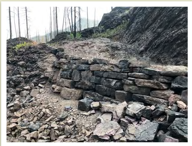
Finished crib wall on Monture Creek Trail #27. (2018)
