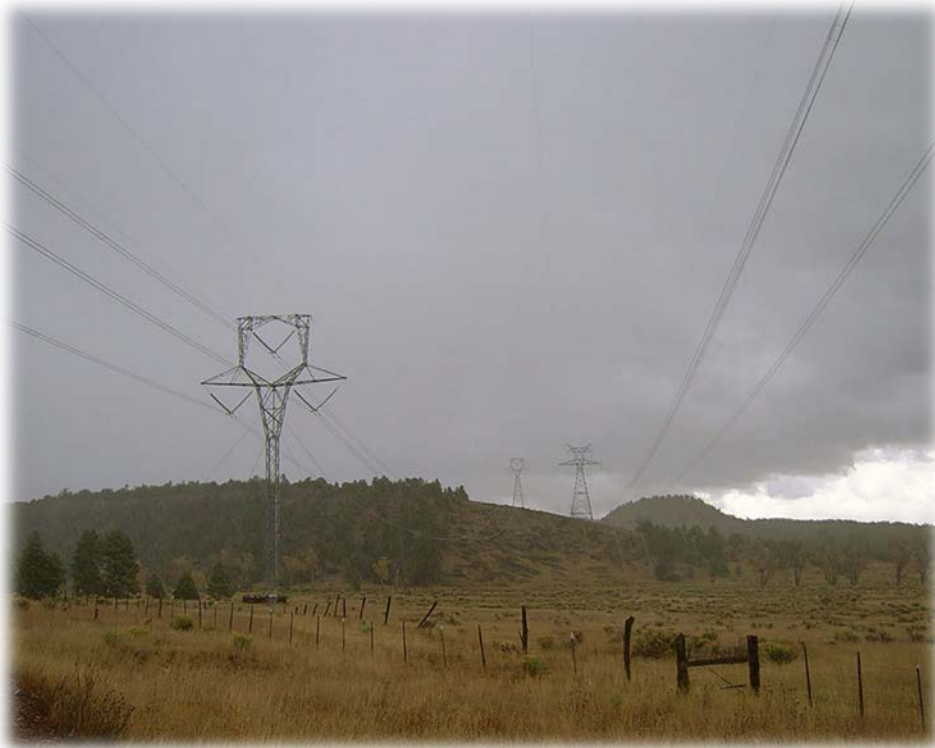
Figure 41 Photo of Large Powerline near Bishop Canyon- Very Low ESI
