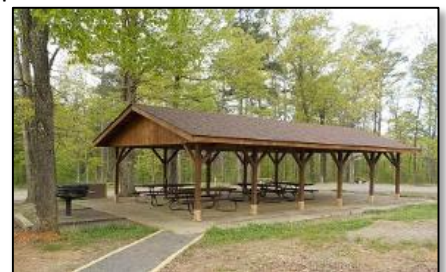
Picnic pavilion repairs and upgrades
