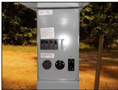
Electrical upgrade at Long Pool
