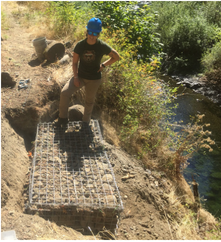
Installing a new gabion box
