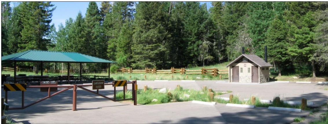
Figure 43. Black Bear Group Campground is an example of moderate existing scenic integrity
