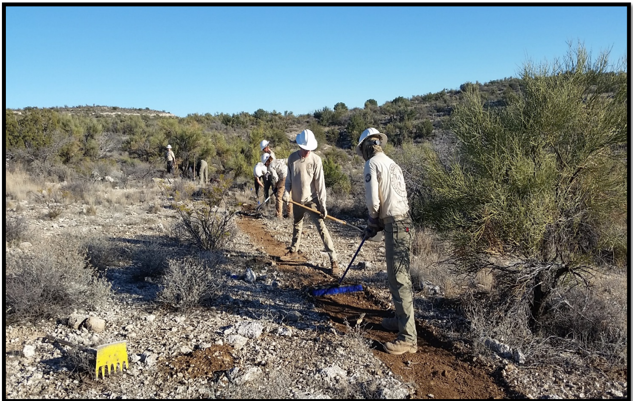
1.5 miles of Grandpa's Wash was rehabilitated and rerouted to move the trail on to a sustainable alignment.
