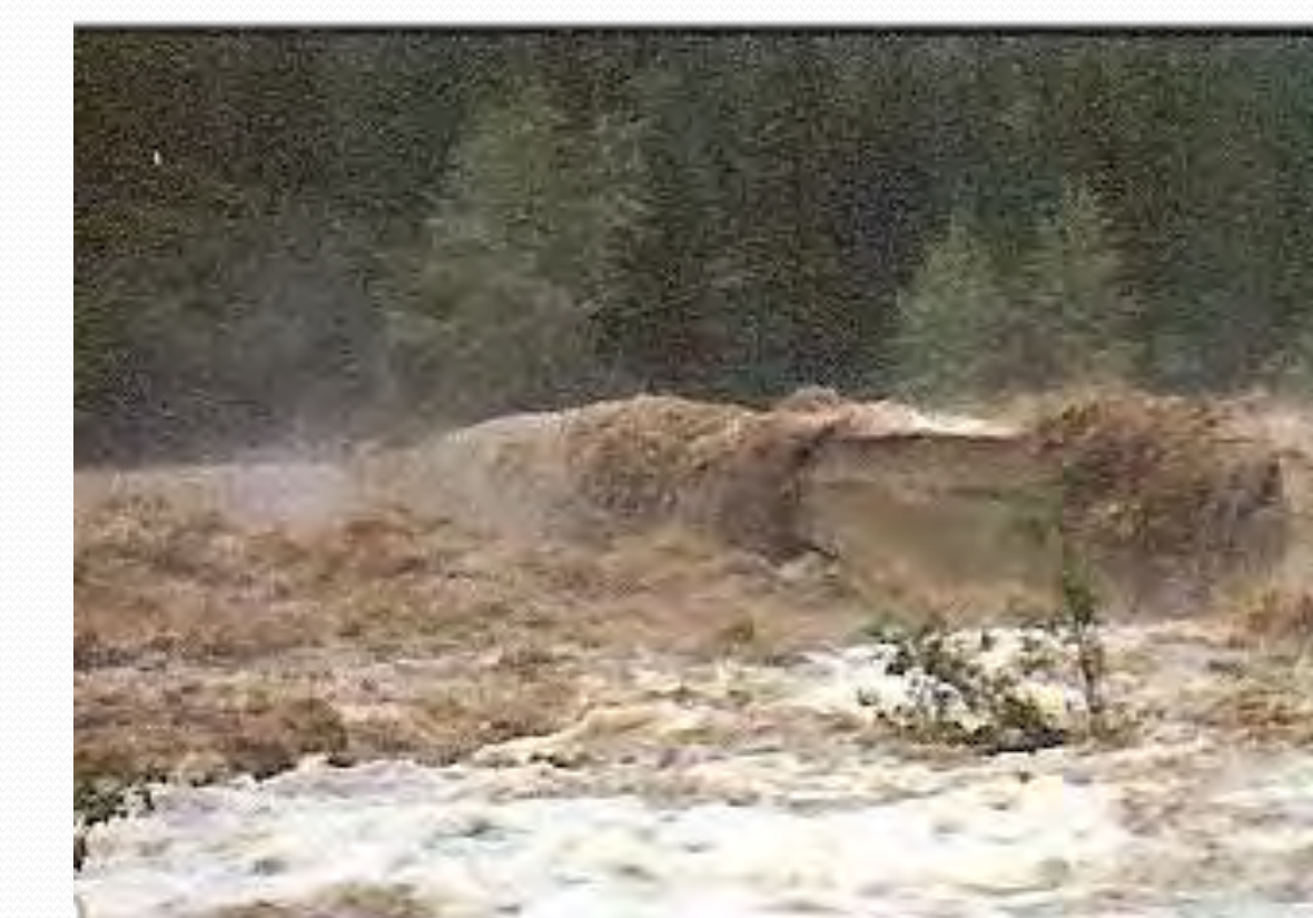
Belton Bridge - 1964 Flood
