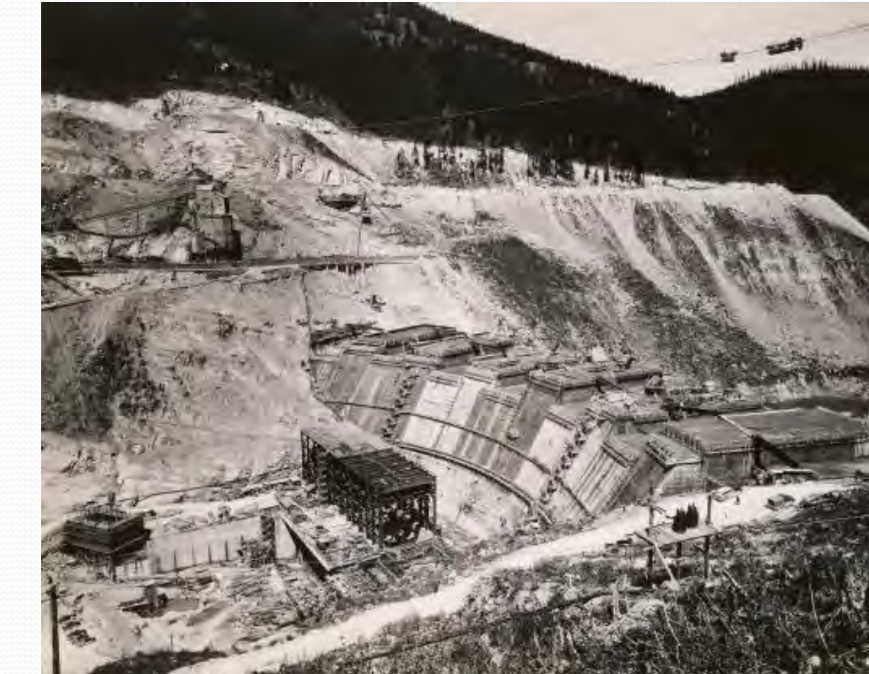
Construction of Hungry Horse Dam
