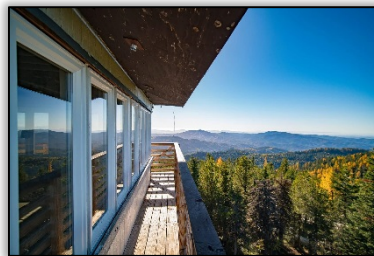
Bald Mountain Lookout: New Catwalks and Lightning Protection
