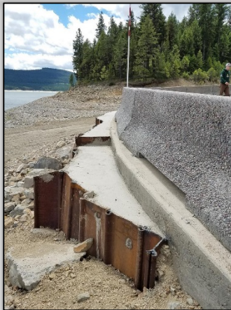
McGillivray Boat Launch after repairs
