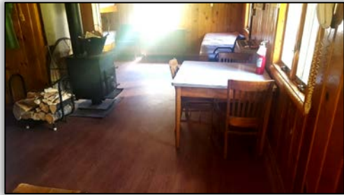
Flooring replacement in the Dry Wolf Cabin
