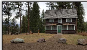
Gravel and barriers at Old Condon Ranger Station
