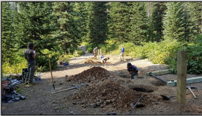
Upper Holland Lake Stock Hitch Rails under construction
