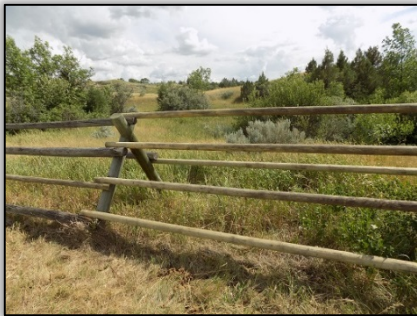
Completed fence repair at the CCC Campground
