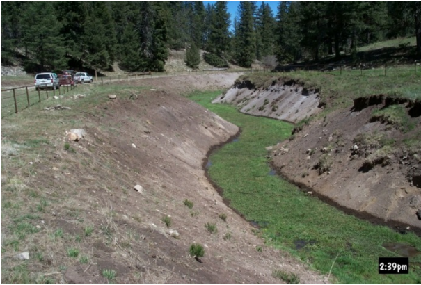
Figure 58. Lowered stream channel along Agua Chiquita Creek, leaving bare banks
