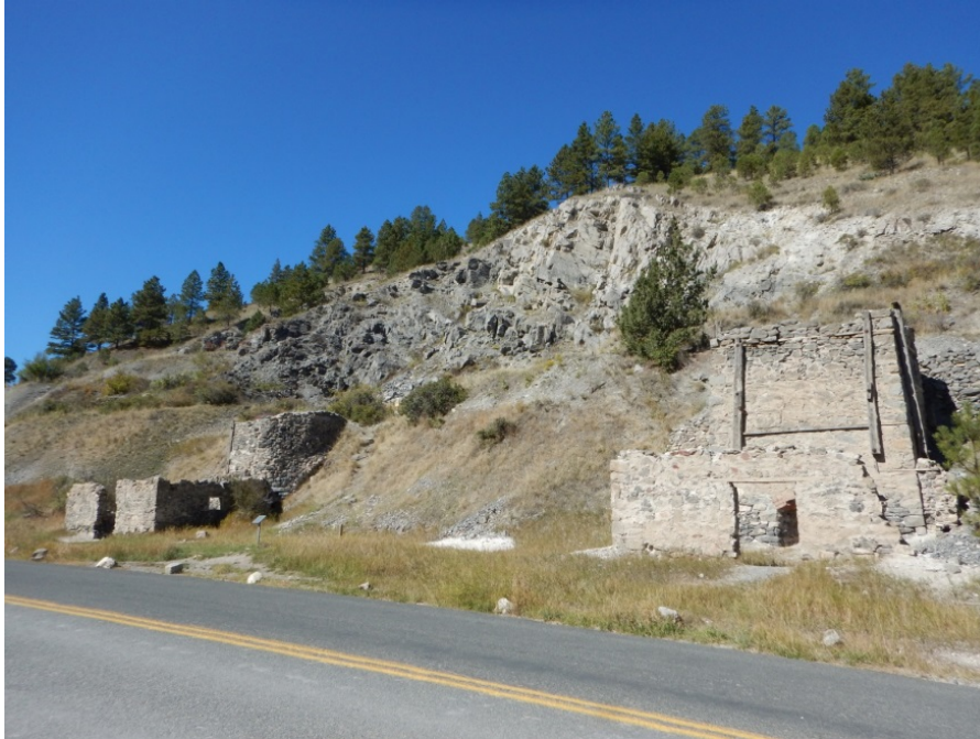
Figure 26. Lime Kiln Remnants in Grizzly Gulch (southeast subarea)
