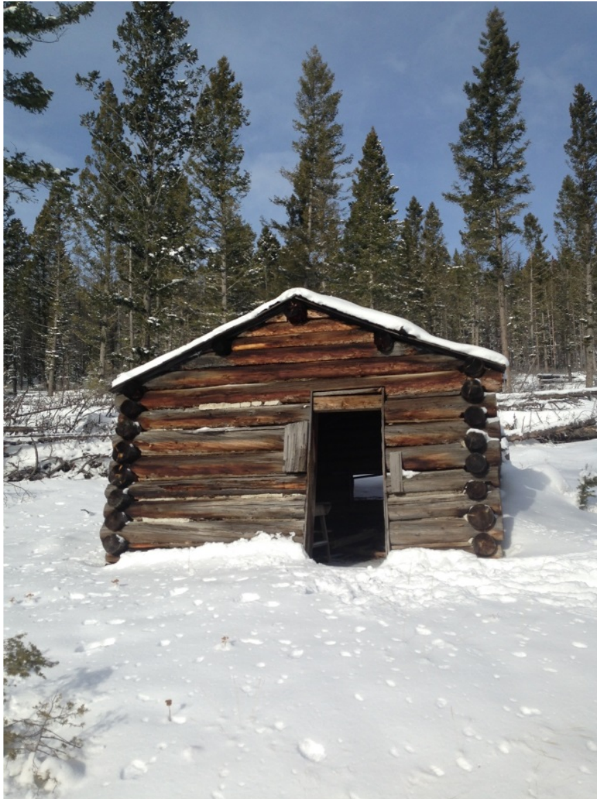
Figure 24. Historic structure (northeast subarea)
