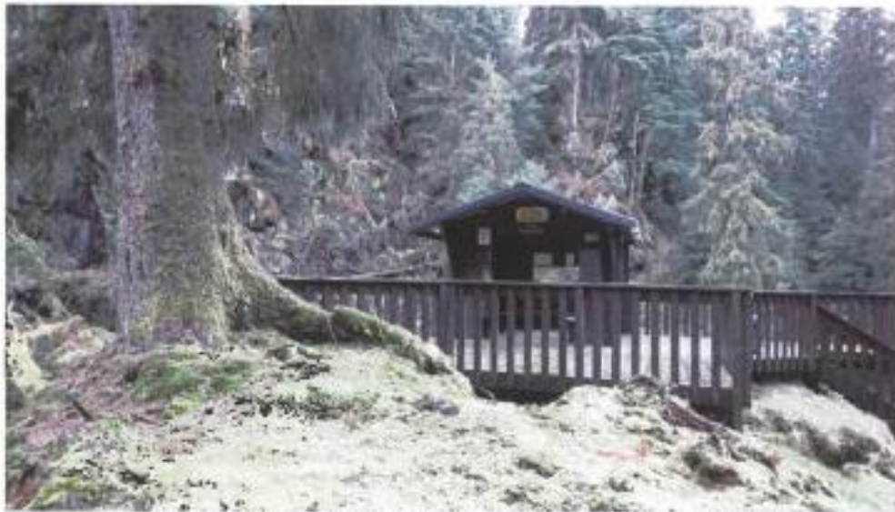
Photograph of the aging Anan Wildlife Observatory structure.
