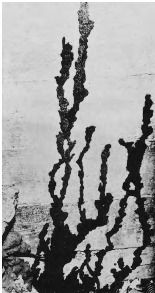
FIGURE 30.—Earthenlike tubes built over cement foundation by western subterranean termite ( Reticulitermes hesperus ).
