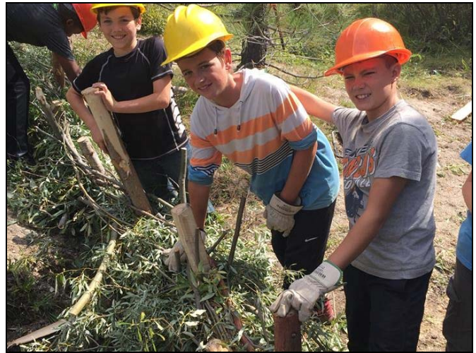
Students add cut willow for the dam structure
