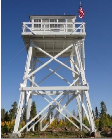
Ute Mountain Fire Lookout Tower
