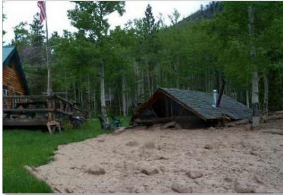
Damage from a debris flow in 2005
