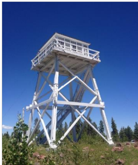
Figure 14. Ute Fire Lookout Tower
