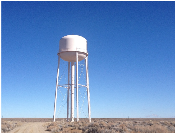
Figure 19. Buckboard water tower
