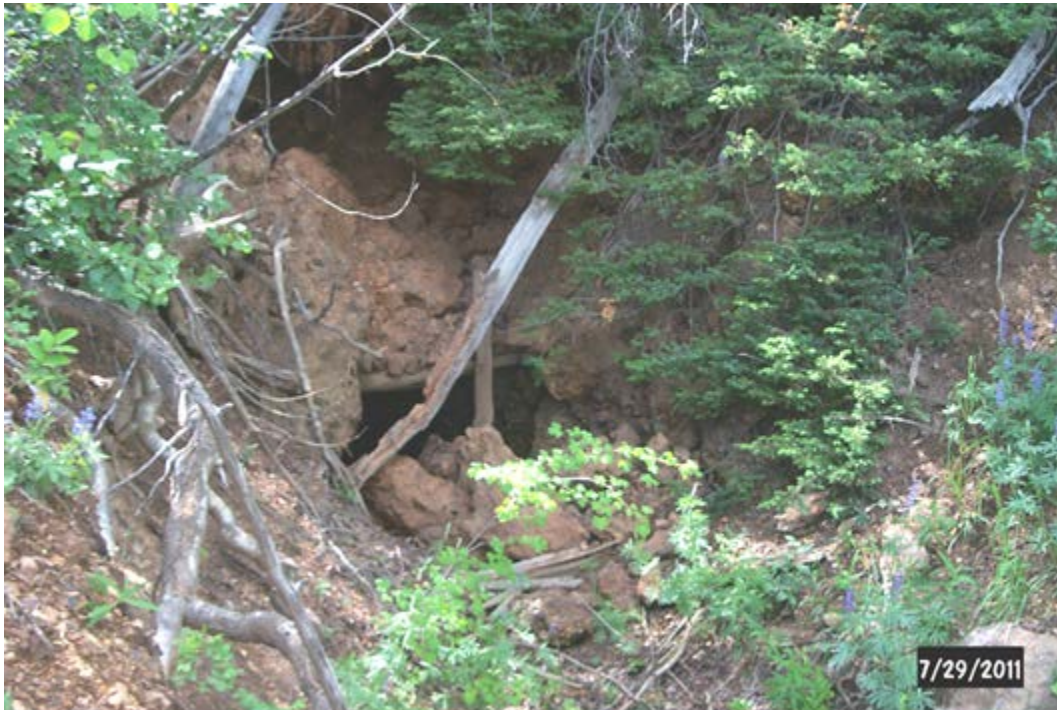
Figure 5. Abandoned mine adit on the Ashley National Forest
