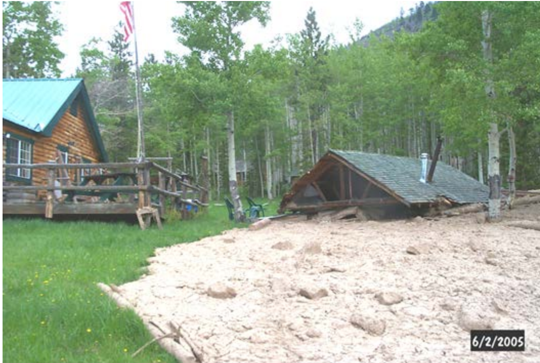
Figure 6. Damage from a recent debris flow on the Ashley National Forest
