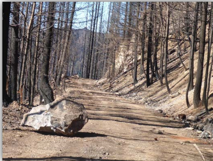
A large rock found on Forest Road 777 illustrates rockfall hazards in the wake of Eagle Creek Fire.
