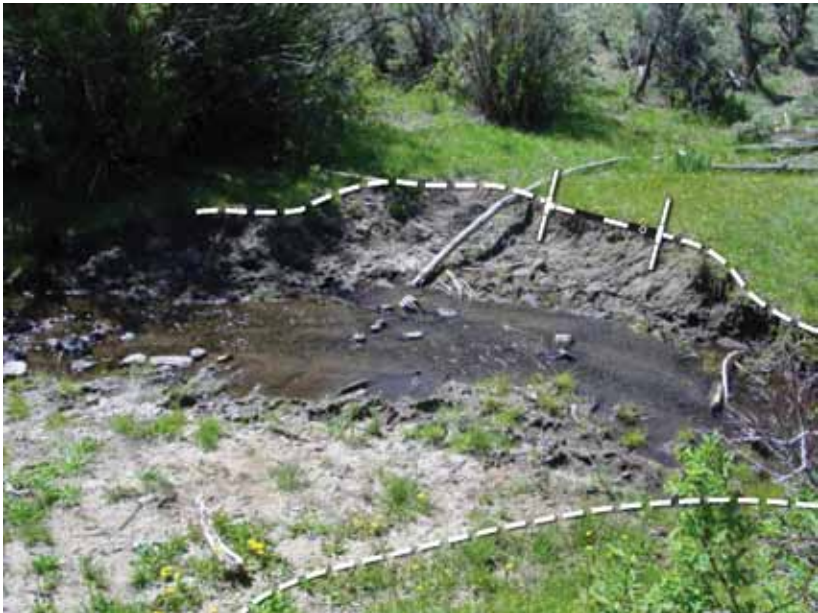
Figure D4. This example is heavily trampled and all five lines intersect streambank alteration. A “5” is recorded.
