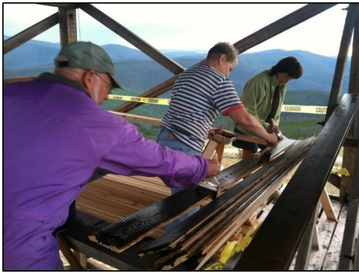
Volunteers working to renovate the Granite Butte Lookout.
