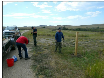
Installing new site posts at CCC campground.
