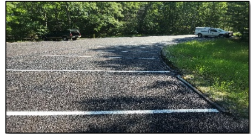
Pavement preservation, Island Lake Day Use Area
