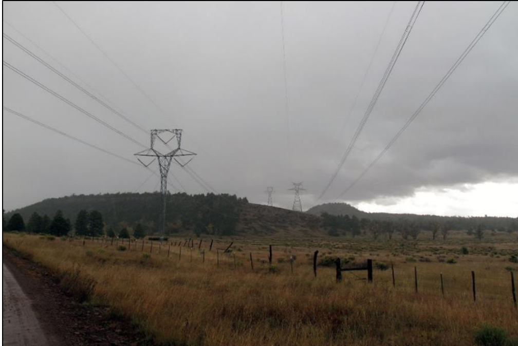
Figure 182. Powerline Utility Corridor in the Foreground Distance Zone
