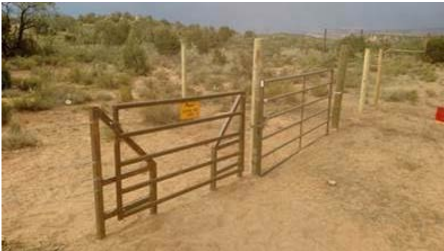
Figure 21. Gate and pass through installed at 9202Y
