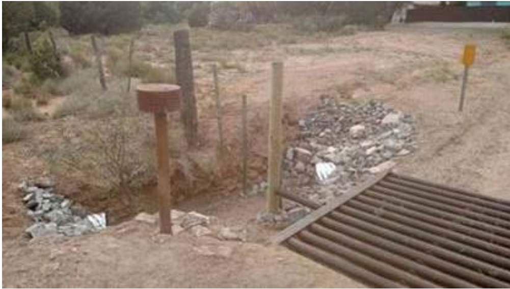
Figure 22. Large gully that was repaired and armored at the 9202Y gate
