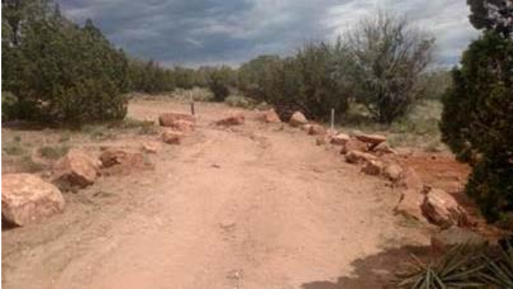
Figure 12. Boulders and carsonite signage placed along FR 9845C to reduce unauthorized motor vehicle use and new route establishment along Dry Creek.
