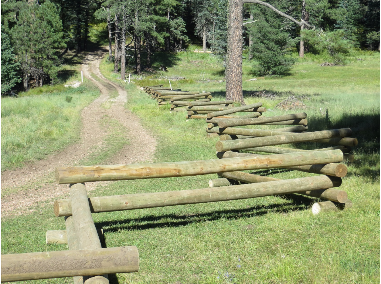
Figure 9. Installed log pole fence to reduce unauthorized motor vehicle use in sensitive meadow habitat at Holder Cabin
