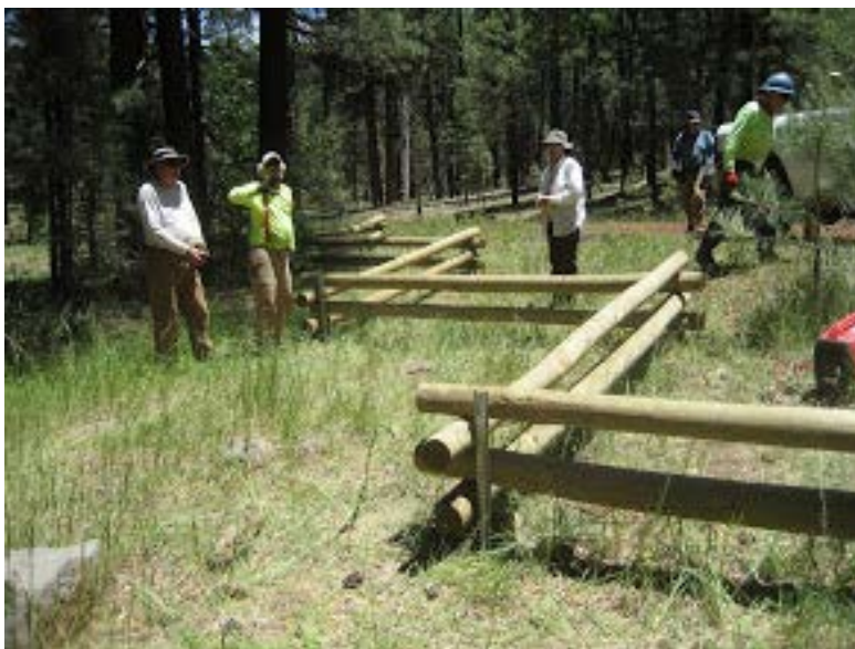
Figure 24. Log pole fence at 9473J
