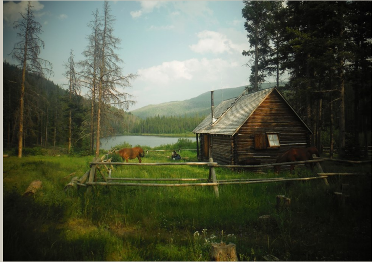
Webb Lake Cabin, where Lincoln Ranger District will be replacing the foundation
