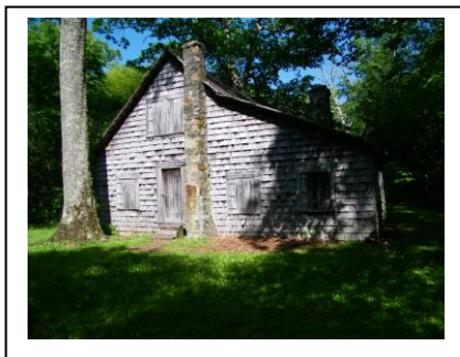
Figure 45. 1916 Wilson Lick Ranger Station Nantahala RD. Shakes cover the Original 1913 log structure.
