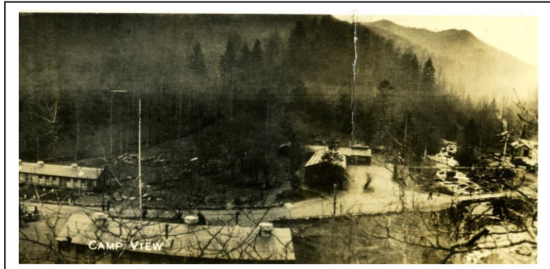
Figure 46. CCC Camp Jim Station Curtis Creek Grandfather RD
